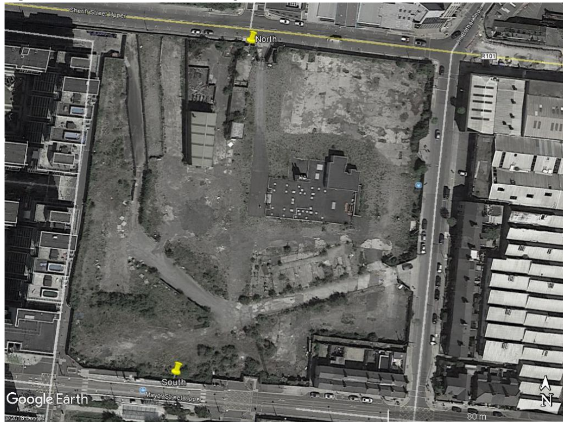
Figure 10.1 Baseline Noise Monitoring Locations
